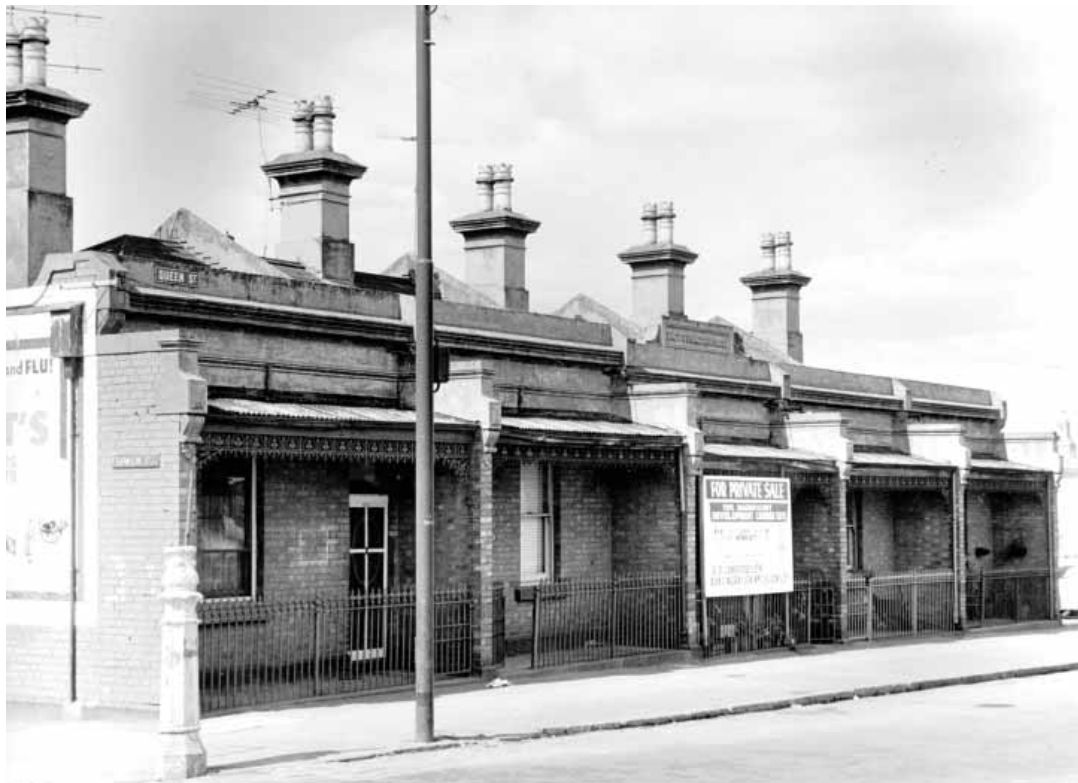
Block of five terrace houses at 408-416 Queen Street, Melbourne (south-east corner of Queen and Franklin Streets), 1960
